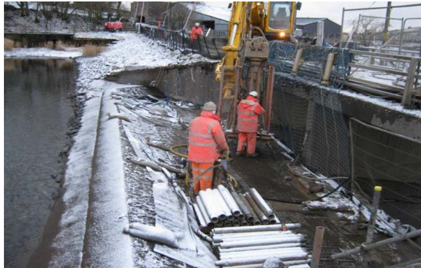
TaM grouting across central spillway, reservoir level maintained
