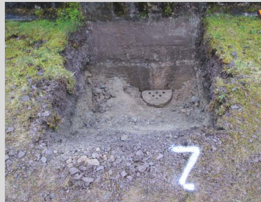
Groundwater monitoring and inclinometer installations
