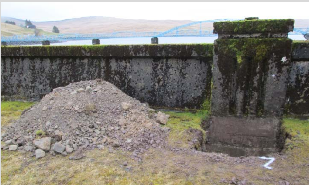
Hand pits & CCTV survey (drainage)
